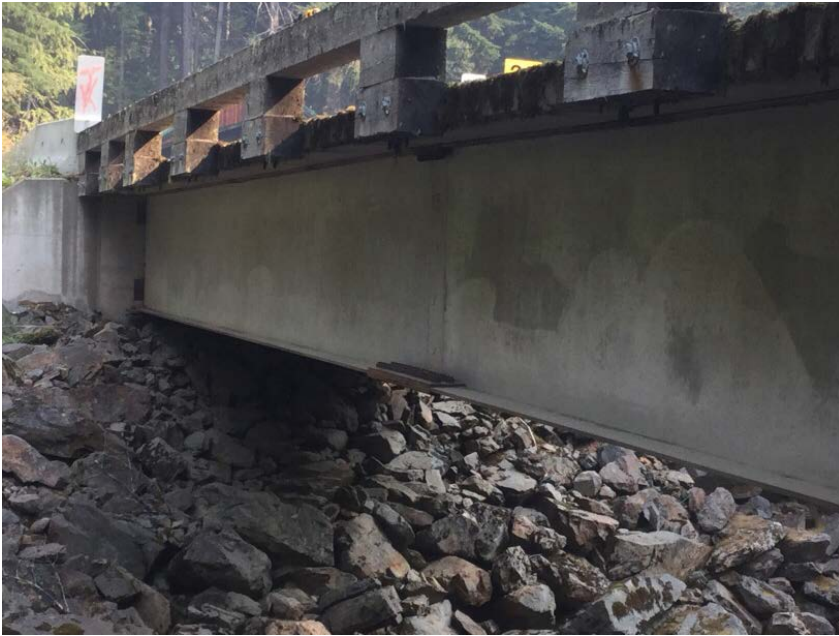
Splice plate on composite girders
