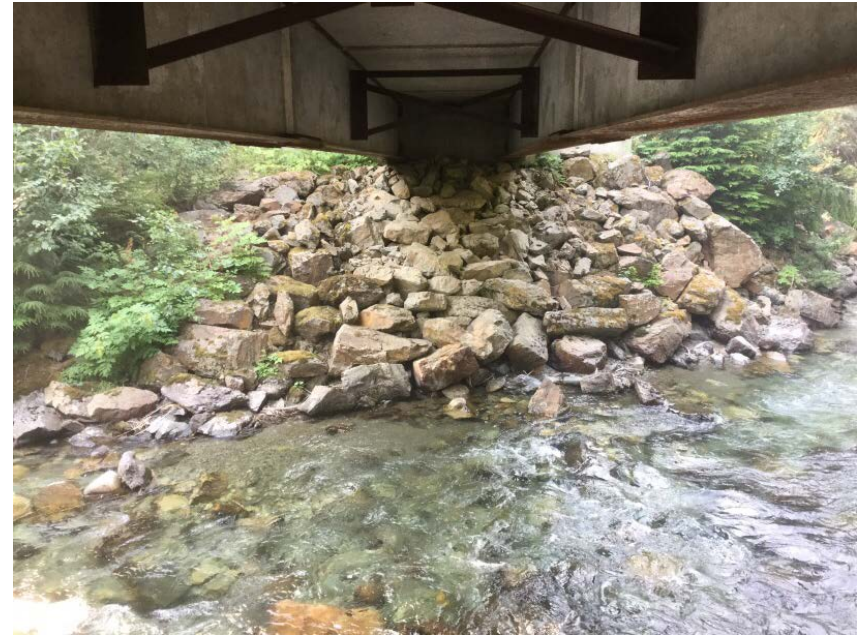
Right Bank Abutment when facing downstream
