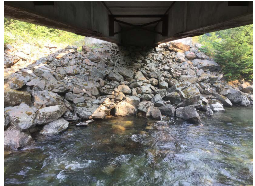
Left Bank Abutment when facing downstream
