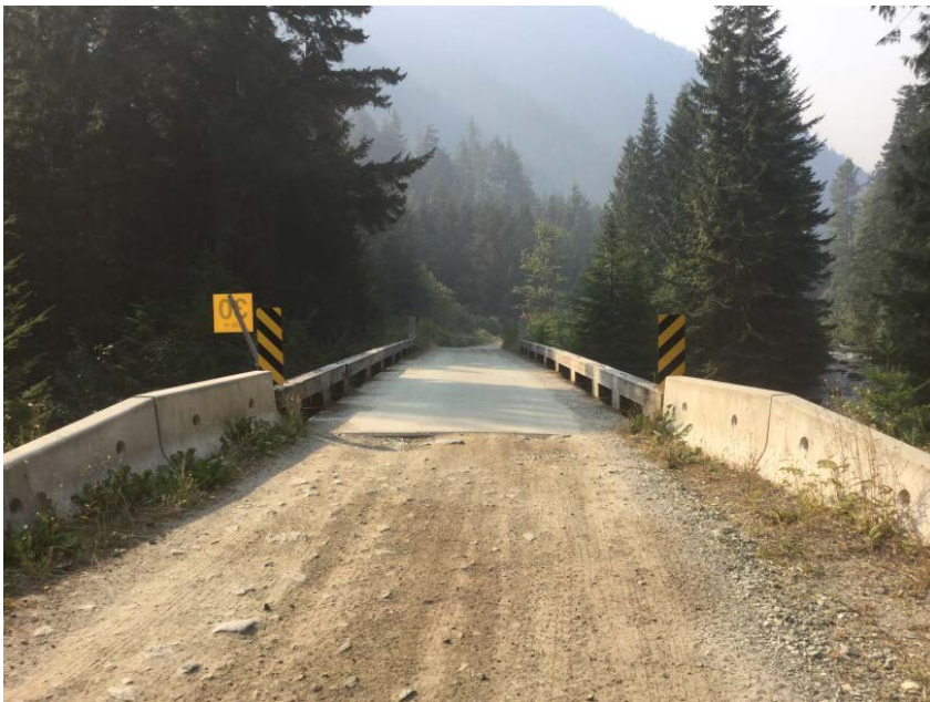
Left Bank Abutment when facing downstream
