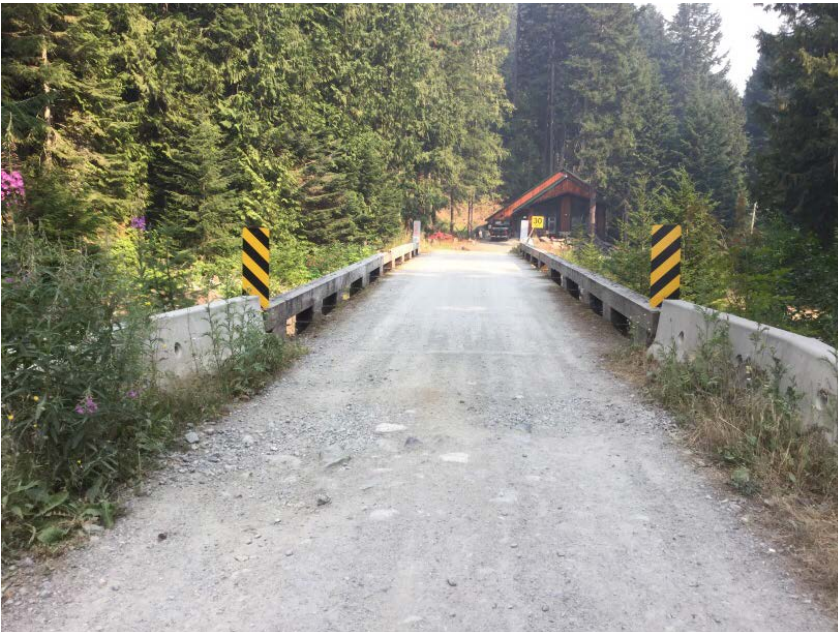
Approach from Right Bank when facing downstream
